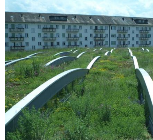
Acoperișuri verzi in Basel (Switzerland)
