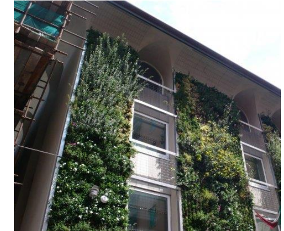
Façade verzi in Genova (Italy)
